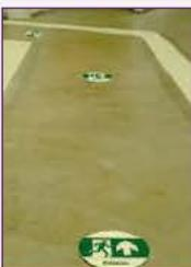
Complements existing wayguidance systems. Suitable for concrete or vinyl flooring and comes with self adhesive backing.
